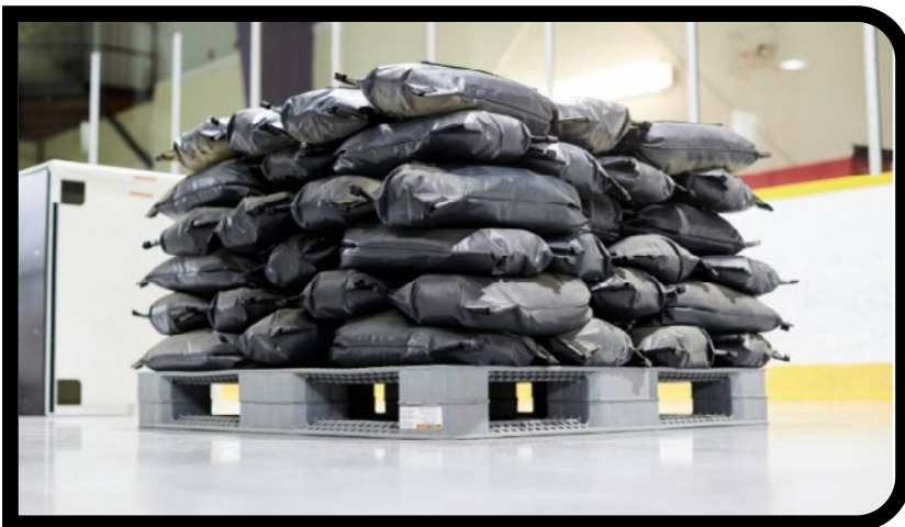
Figure 41: Alternate layers of sandbags
