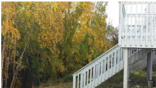
Exterior View at Back/Treed Area
