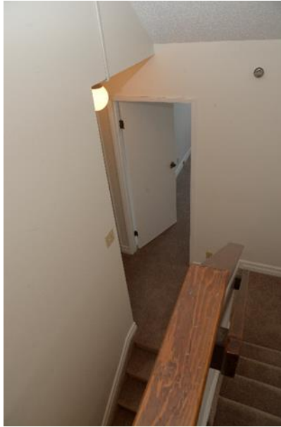
Staircase From 3 rd Level
