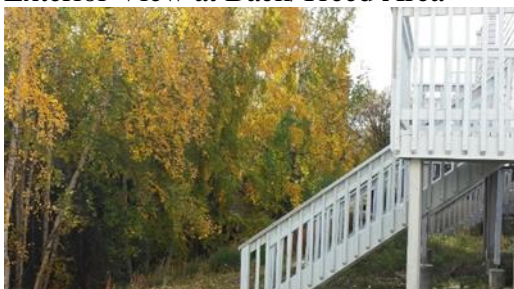
Exterior View at Back/Treed Area
