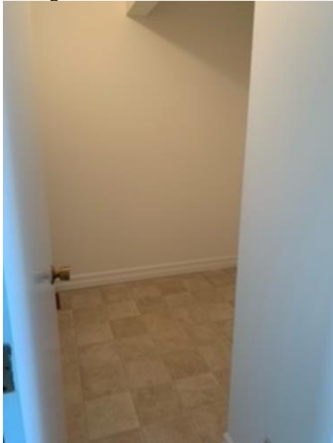
Storage Room 2 nd Floor
