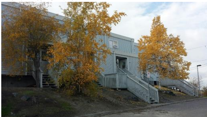
Front Exterior View
