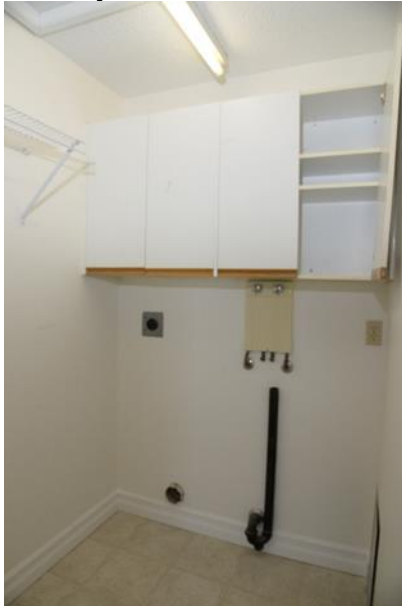
Laundry Room 2 nd Level
