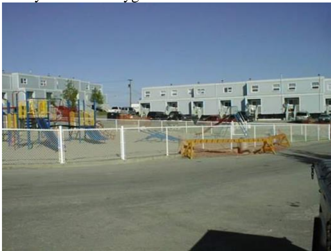
Lanky Court & Playground Area Front Exterior
