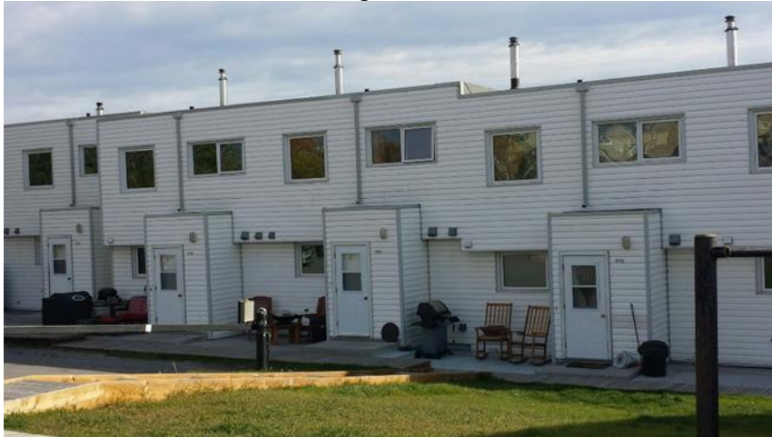
Exterior View from the Parking Area
