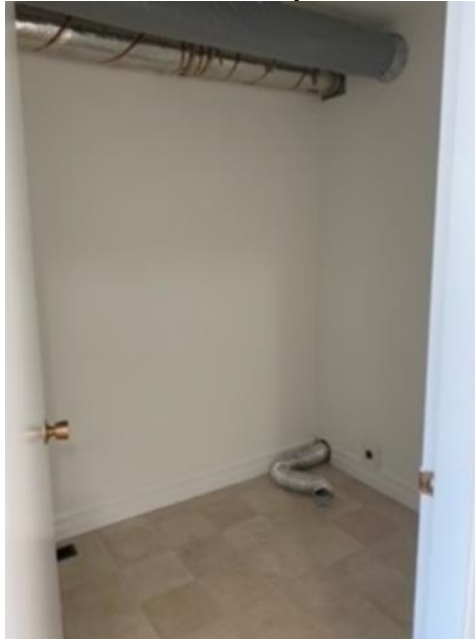
Main Floor Laundry Room
