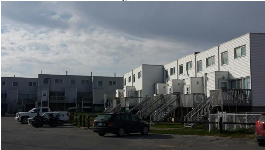
Exterior View from the Parking Area
