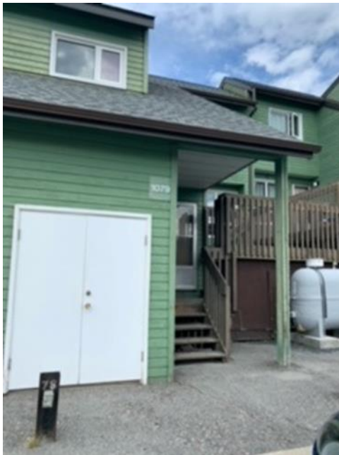
Exterior View at Front
