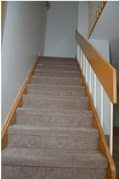
Staircase to 2 nd Floor
